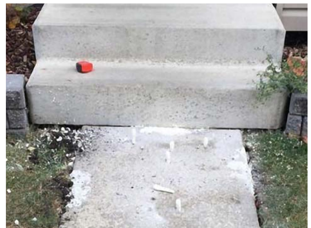
ECOTITE SJ Slabjacking After
