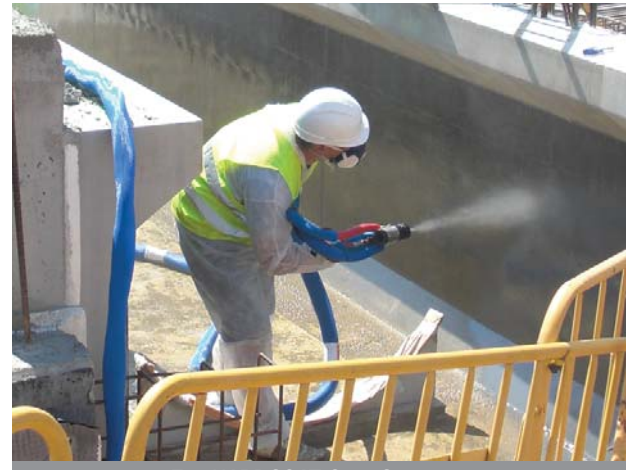
Z-7 HARDCOAT Over Concrete
