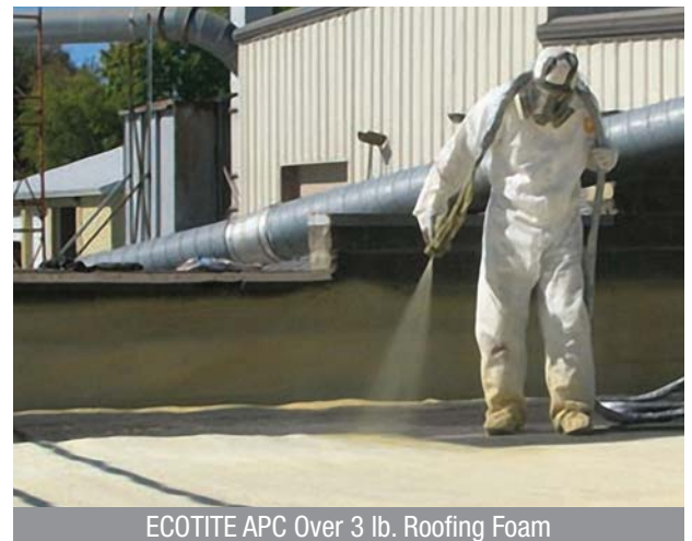
ECOTITE APC Over Steel Roof Deck
