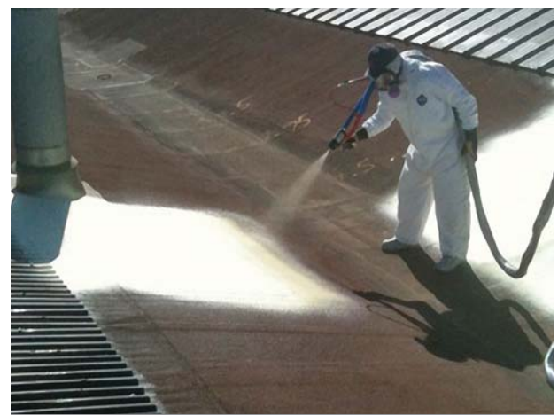
ECOTITE 3.0 Roofing Application
