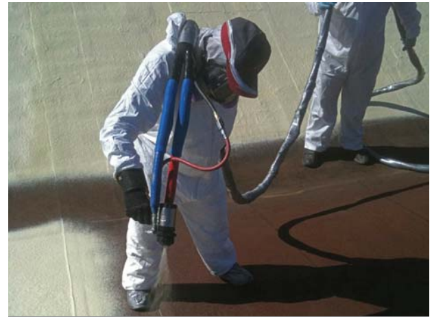
ECOTITE 3.0 Roofing Application
